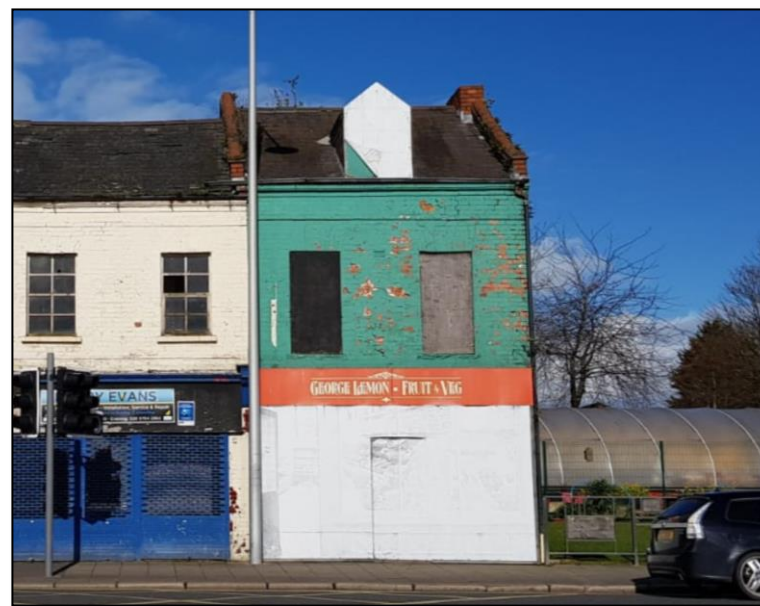
Figure 4 - Photo of existing building
