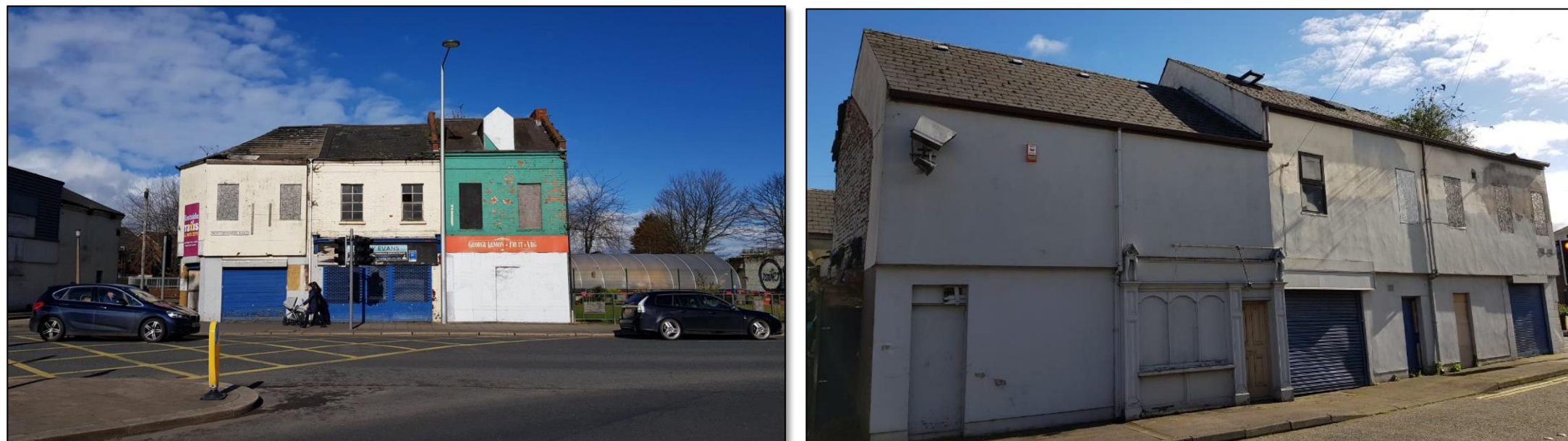
Figure 8 - Current photos showing some remedial work carried out since the fire
